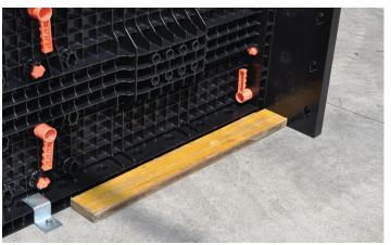
The anchoring to the ground is useful to avoid lifting of the formwork and it is done using metal or timber brackets.
